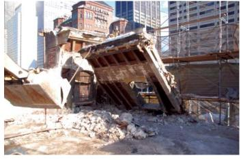
Shoring is typically used on all floors as the work proceeds. The purpose of shoring is to increase the live load capacity on the deck that is currently being worked on and to give the structure additional support. As each floor is demolished, shoring is removed.
