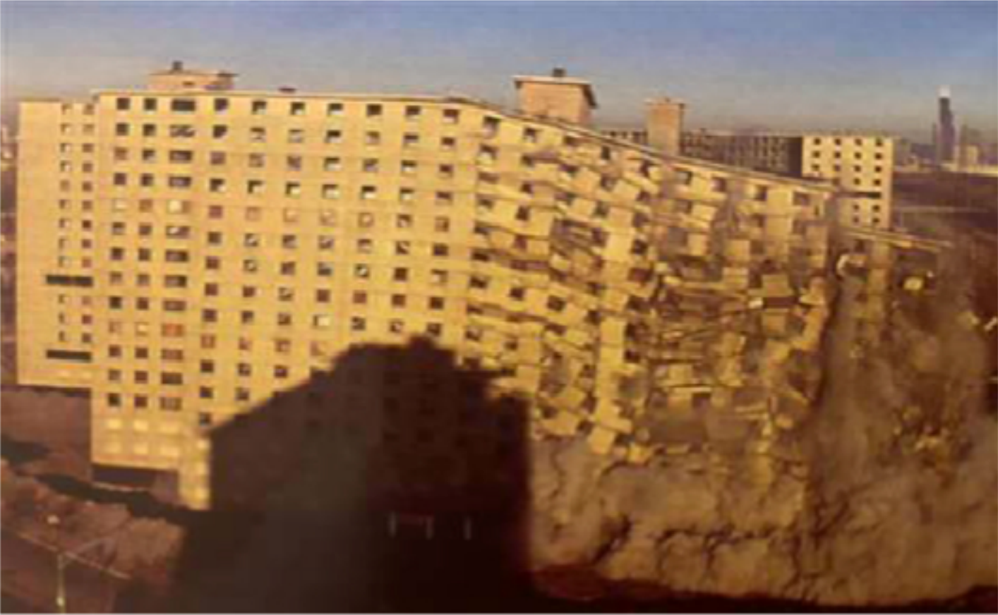
CDI's loading crew placed 830 lb (376 kg) of explosives. (PHOTO: Brandenburg/CDI)
